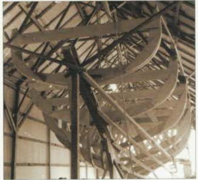
Scimitar's hull takes shape in 1957 with the vertical moulds and the lengthwise ribbands in place - photo courtesy of Barry Purcell
