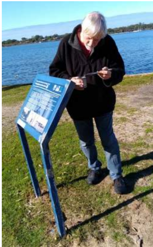
Touching up paint on interpretive sign after removing rust.
