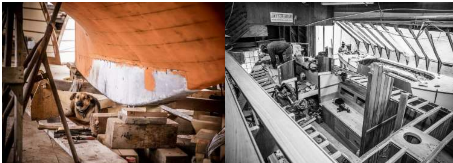
The G&B boat yard supervisor signals official approval of the keel of the Nat Benjamin design 86 ARTEMIS In the front shed Design 86 Artemis. South to her is another close to completion Design 1
